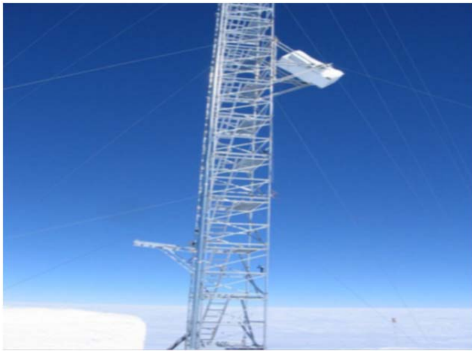
Fig. 1 - Radomex installation on the US tower. The Panasonic CF30 Laptop is inside the box of Radomex
